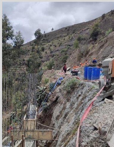
Construction of a retaining wall in the Peasant Community of Colca
